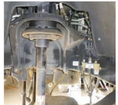
Figure C: Reinstalling strut with TRAXDA strut cap
